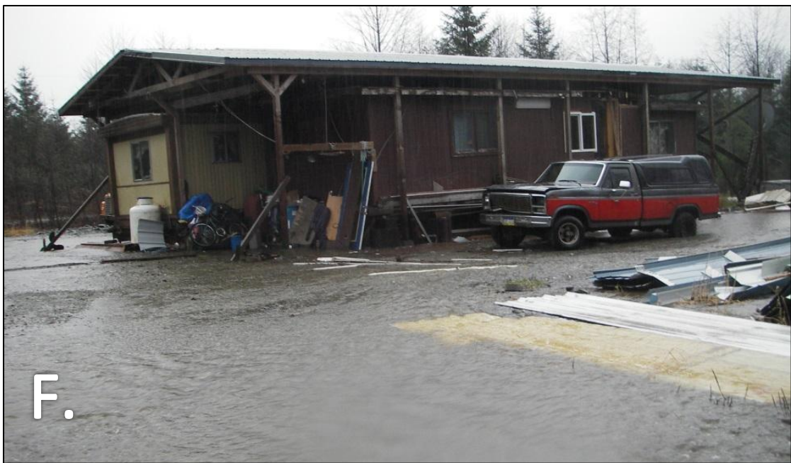
Figure 5. E) Culvert outlets at the Klawock-Hollis Highway during a flood in 2005. F) Flood waters on the property just downstream and to the south of the culverts. Photos courtesy of Mark Minnillo.
